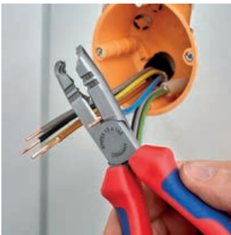
Cutting when shortening single conductors
